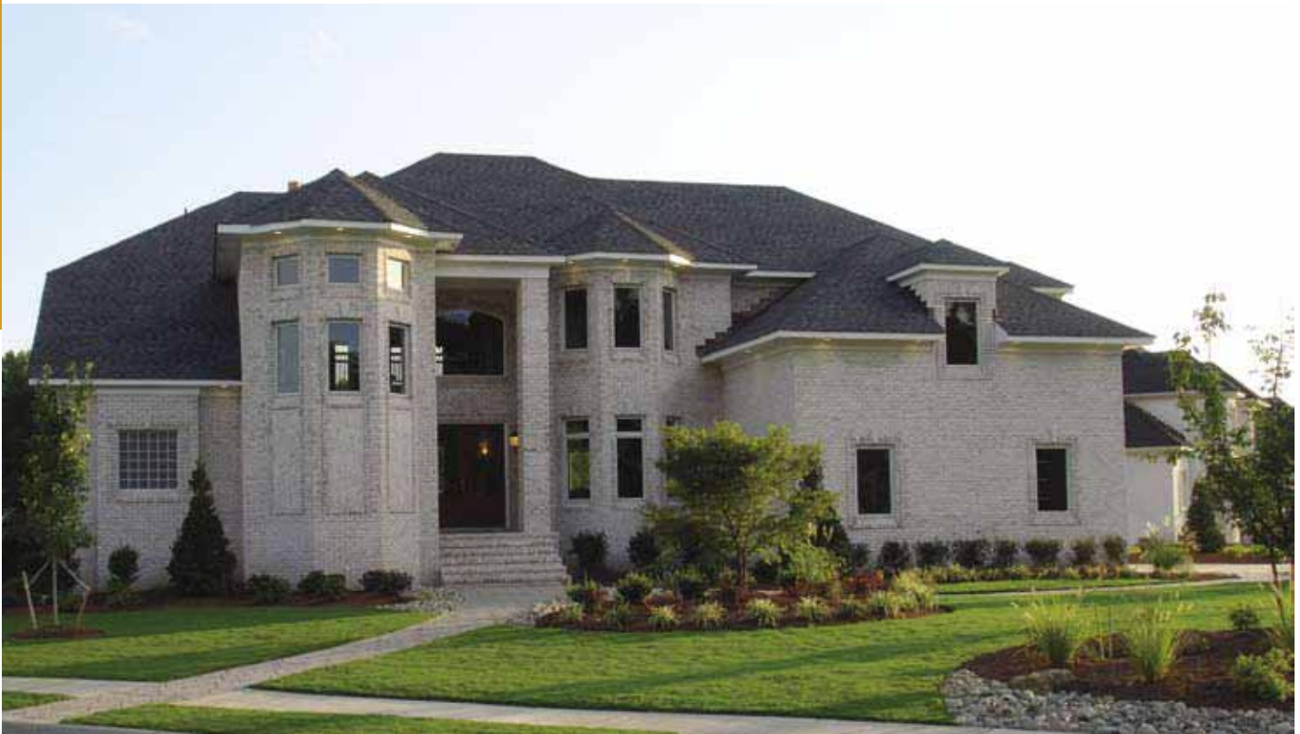
The first EarthCraft House™ in Tidewater, Virginia, built by Miller Custom Homes.
