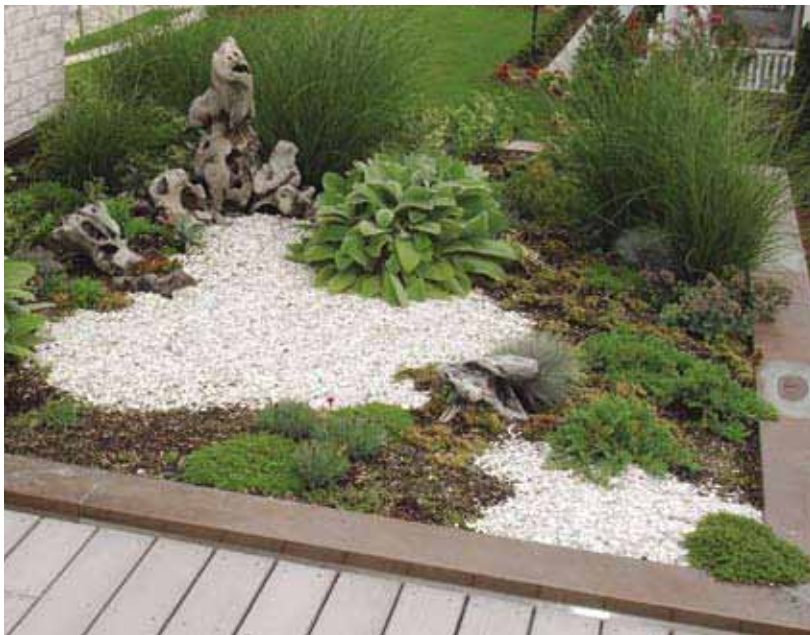
Living green roofs are covered with soil and vegetation to be enjoyed as an expansion of the home’s yard areas. This type of roof reduces storm water run-off and aids in filtering pollutants out of the air.
